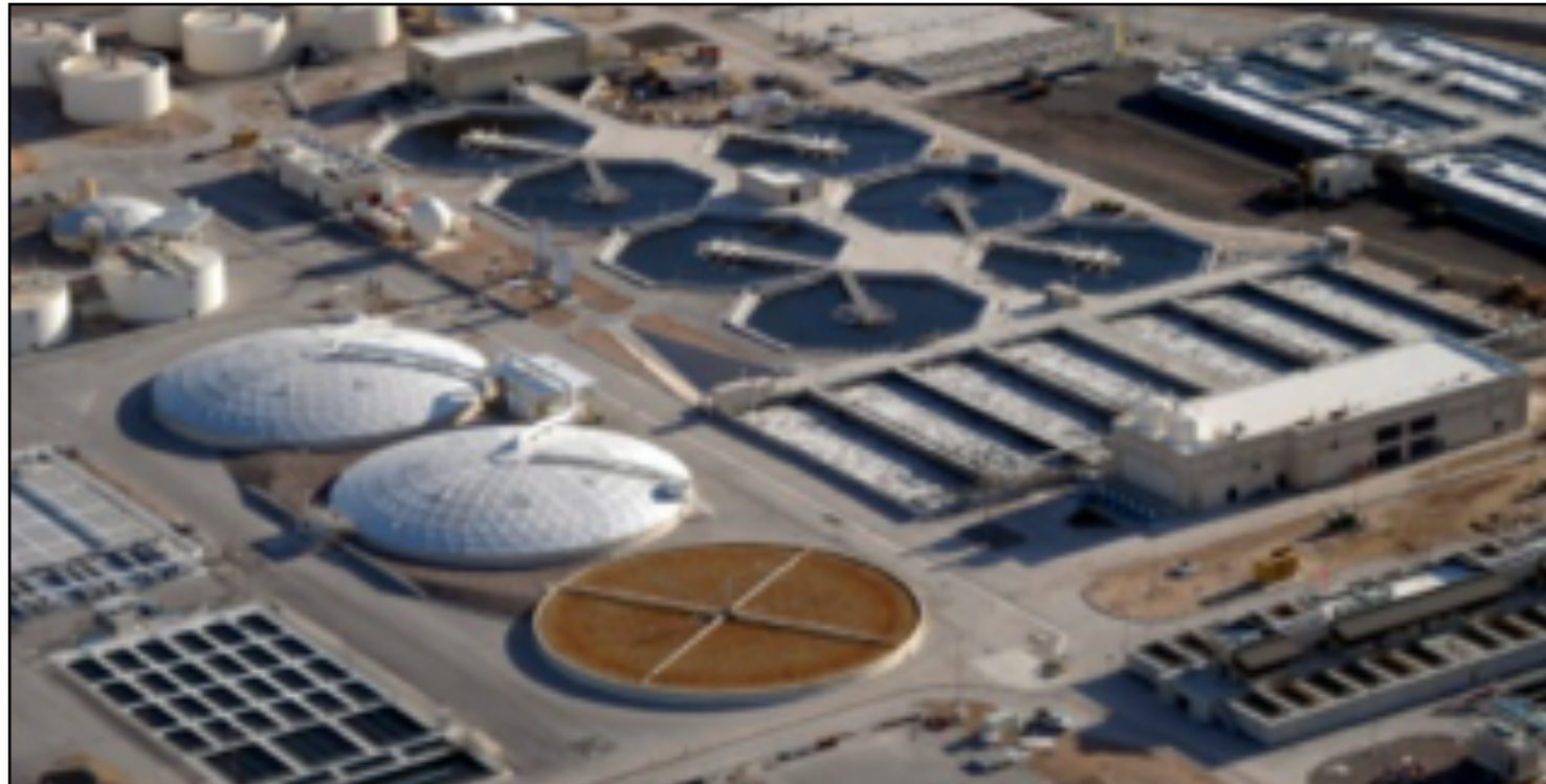
Figure 1.1 AERIAL VIEW OF A WASTEWATER TREATMENT FACILITY
